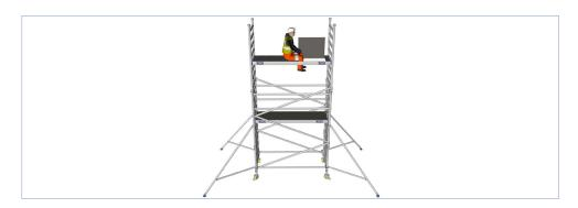
1.30 Put the handrails in the correct place. The first will be placed approx. 250mm from the platform, (the 2nd rung above the deck) and then again at 500mm (the 4th rung above the deck).
