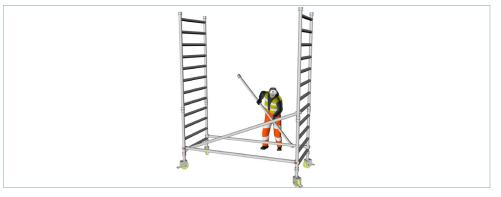
1.11 Clip the diagonal braces onto the lowest rungs.
